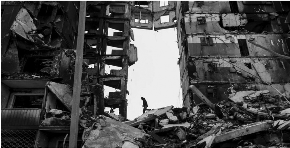
Apartment building in Ukraine destroyed by Russia
